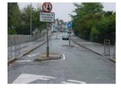
2. Speed tables (plateaus). These are okay at junctions and crucial points but should not be placed in a great series. They create less bumping and offer the possibility of a raised crossing point. However, they also cause the most damage to buses.
